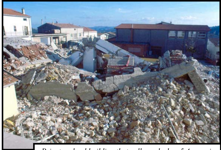
Private school building that collapsed when 5.4 magnitude earthquake struck San Giuliano Di Puglia in Italy in October 2002
